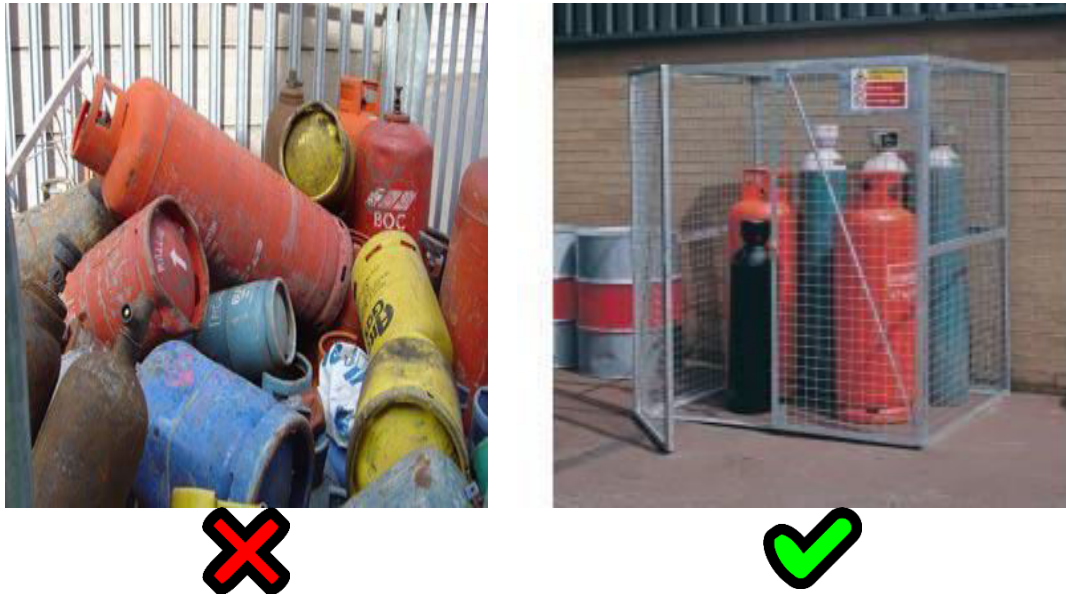
Fig. 2. Examples of the incorrect and correct outside gas cylinder storage (correct storage must be locked when not in use).
