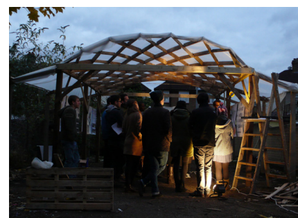
Unit 6 built a lamella roof on a redundant garden site on the Isle of Dogs for social housing group East End Homes.
