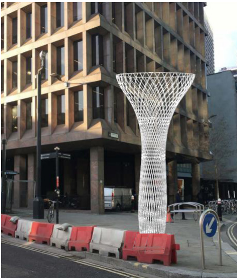
Ventilation Casing, Aldgate Square
