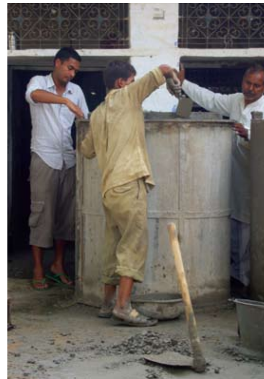
Student constructing prefabricated septic tank, Kuchhpura, Agra. Photo: Bo Tang
