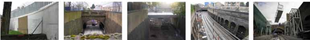
Reconstituted brick in retaining wall
